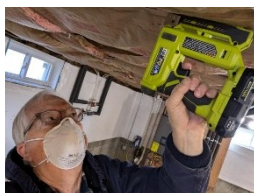
Chip Thurlow Stapling Insulation
