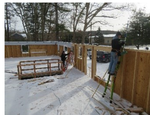
John and George working on installing the vapor barrier
